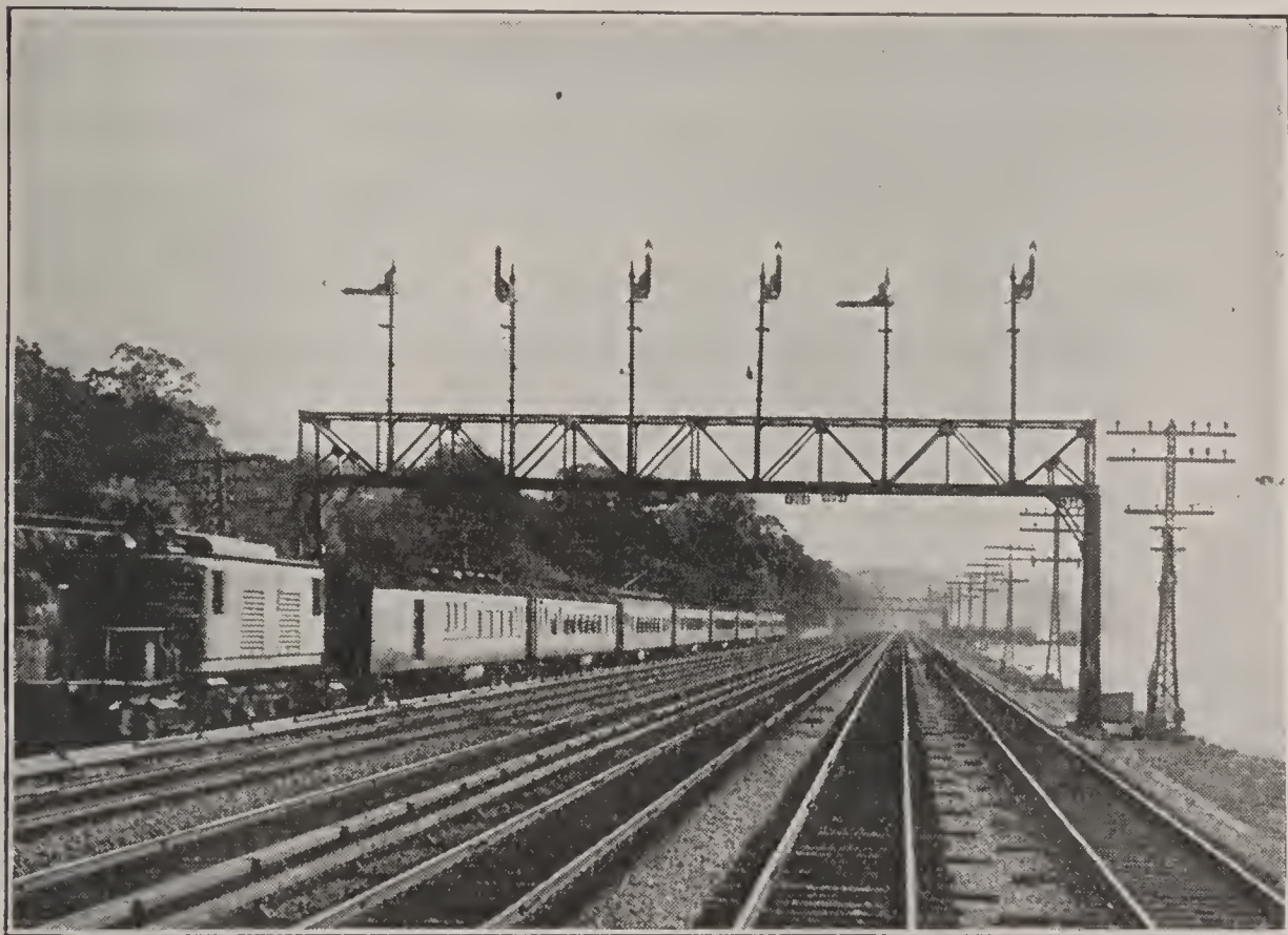
The Block System of the Modern Railroad is Controlled by the Telegraph.
